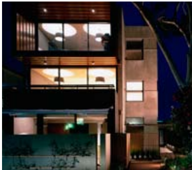
36 Wynnstay Road, Prahran 8 apartments, 2004
